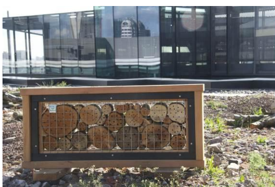
Figure 1: An example of a bespoke insect/bee wall (The Green Roof Consultancy).
