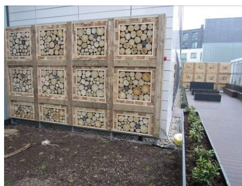
Figure 2: An example of a large insect wall on a green roof (The Green Roof Consultancy).
