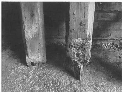
Figure 1. Rotten bases on two of the fence posts
