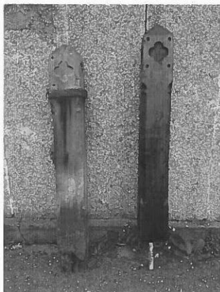
Figure 4. Right: restored test post, left: unrestored post for comparison.
