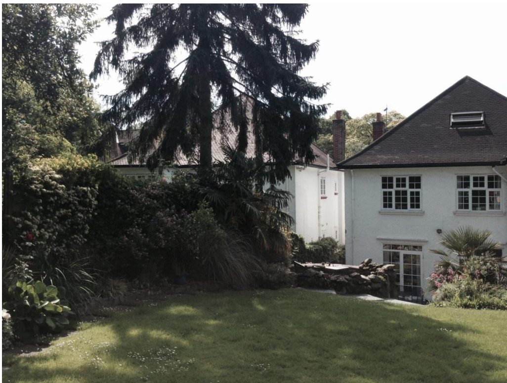
Photo 4: View of rear elevation and boundary with No. 6 Holly Lodge Gardens
