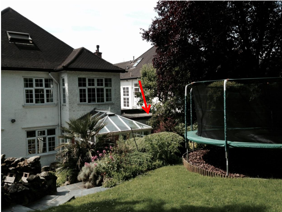
Photo 3: Existing rear elevation and roof of rear conservatory visible on boundary with No. 5 Holly Lodge Gardens. Arrow shows location of second set of doors to be replaced.
