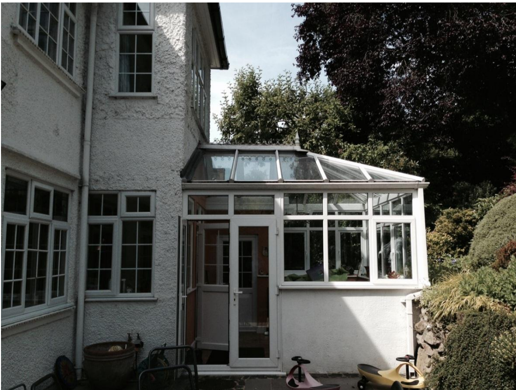
Photo 2: Existing rear conservatory
