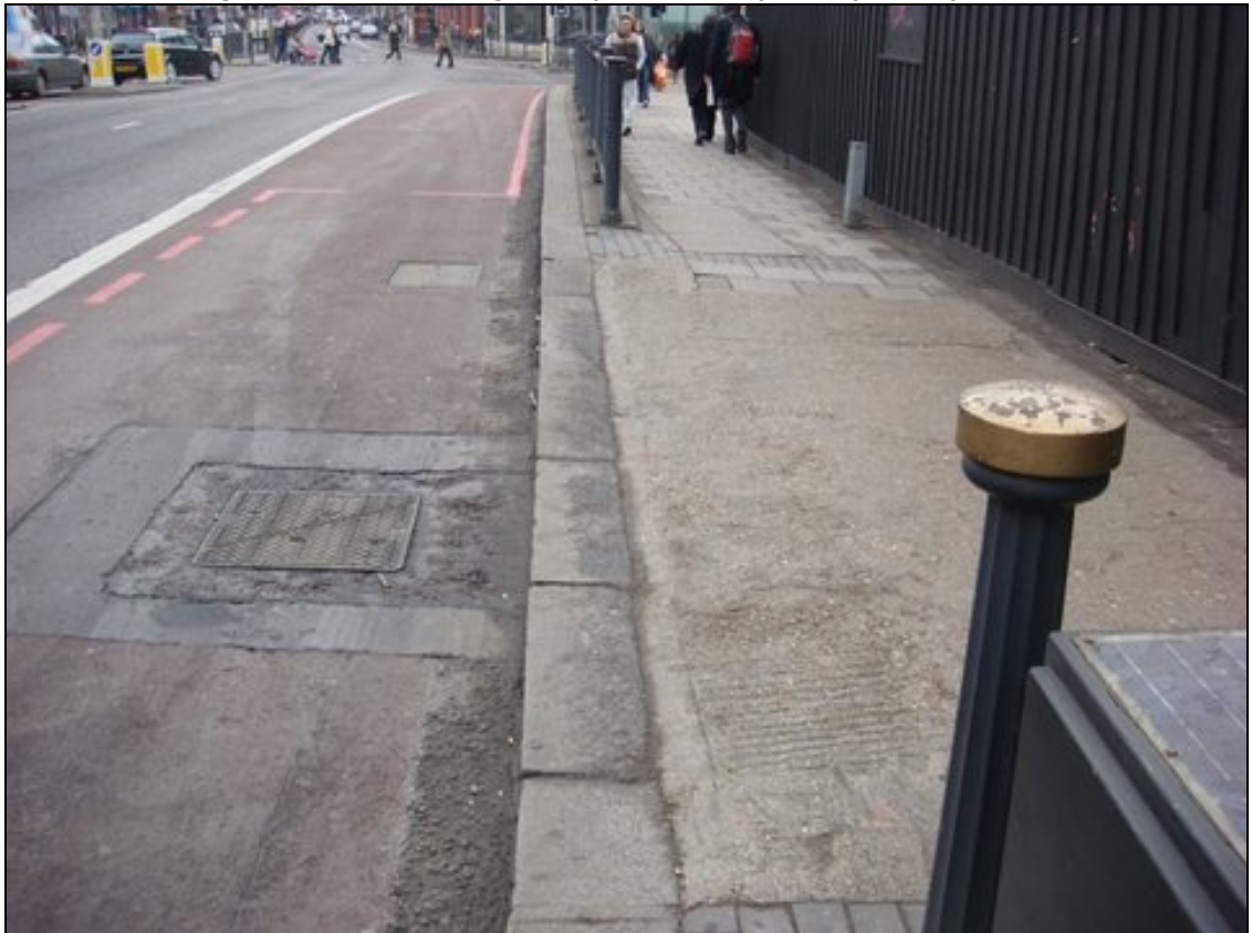
Photo 2: Building Access Point looking south from Finchley Road footway
