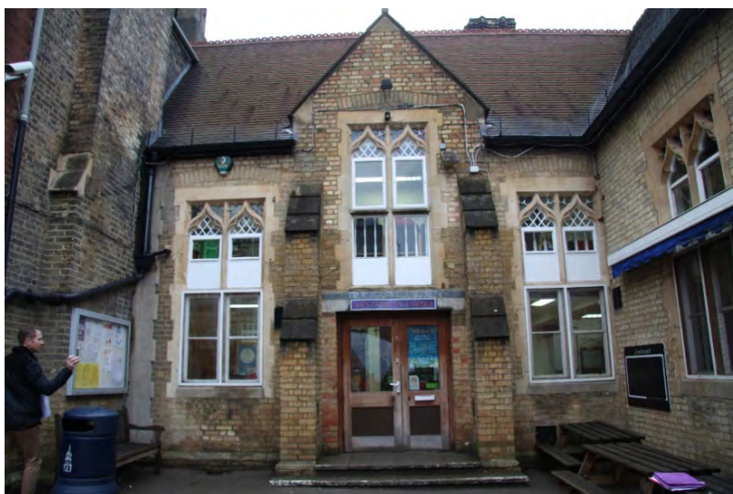
South elevation of school showing main entrance doors, inserted in place of the original windows in the 1970s
