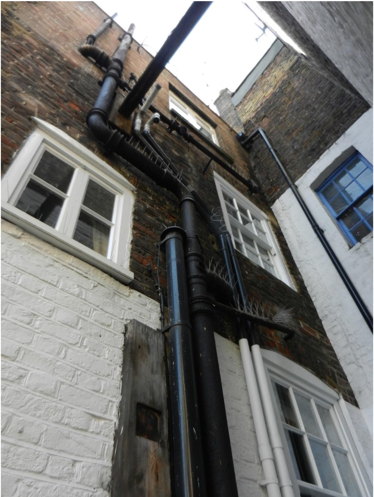
Rear elevation looking up at first to third floors
