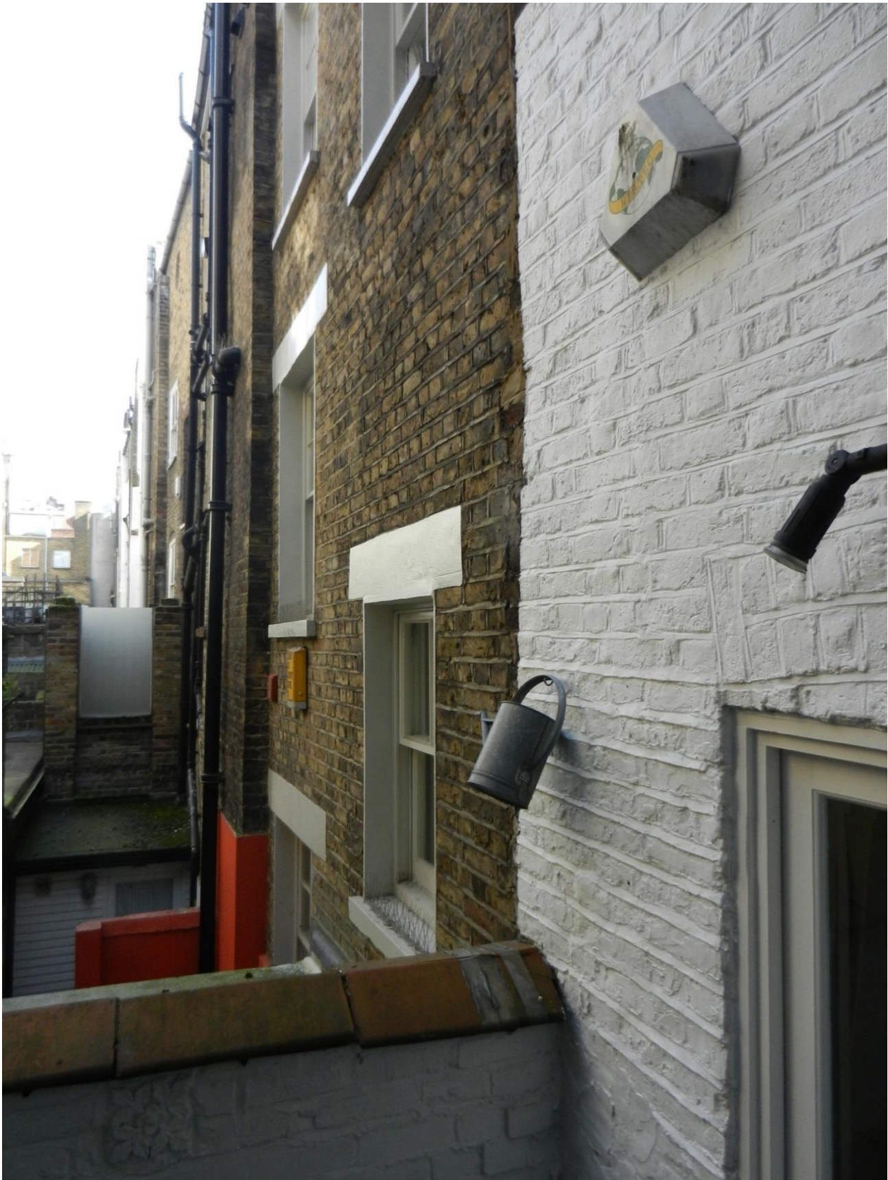
Rear elevation looking east towards 12 Colville Place
