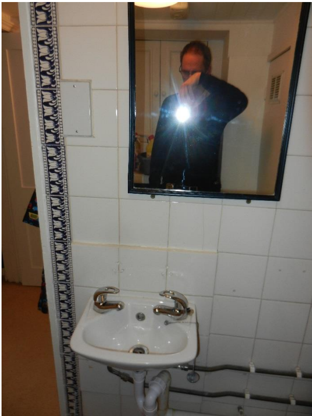
Rear WC looking towards front of house and lobbies
