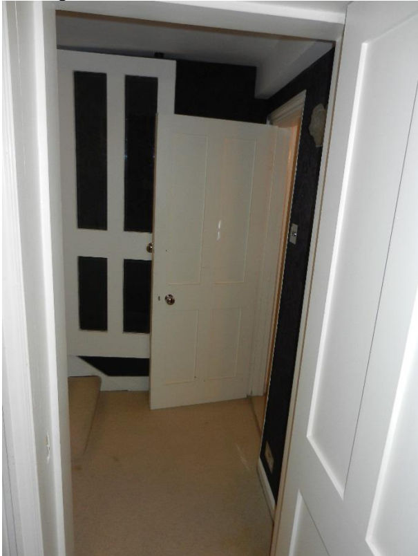
Looking towards party wall with 12 Colville Place
