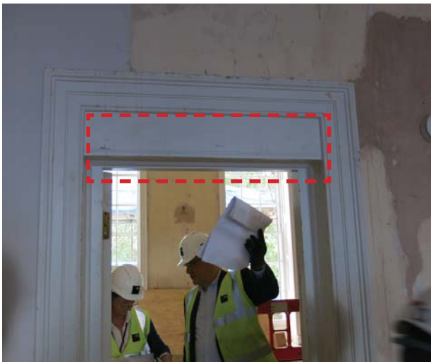
C. First floor door (FD.11). Frame and door head to be removed and reinstated to original proportions
