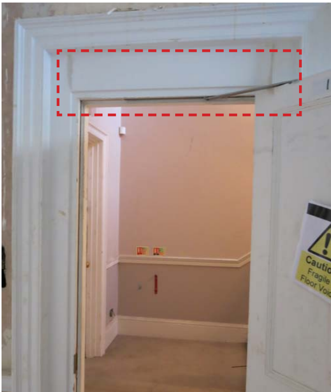
B. First floor door (FD.08). Frame and door head to be removed and reinstated to original proportions
