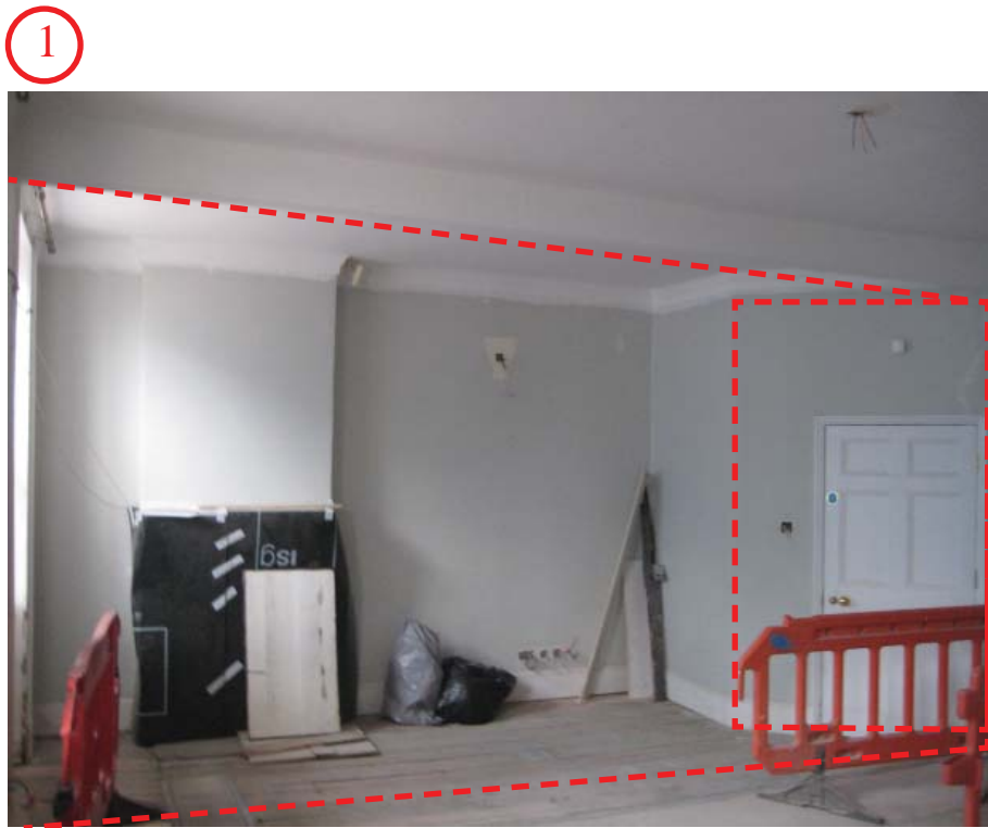
New Partition on line of existing downstand to subdivide office
