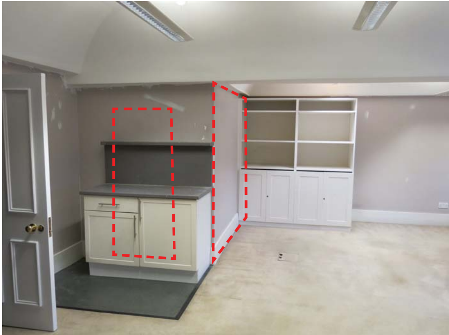
Partition removal and new door (Seen from T8. Room 15.12)
