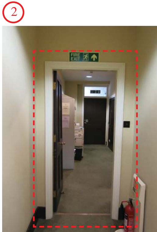
Existing BD.03 to be relocated, partition removed. (Seen from B1. Lockers)
