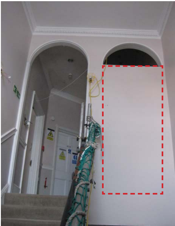
A. Second floor stairway arch at no. 15 to be reinstated to match original at no.16.
