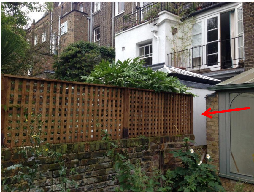
Photo 3: Boundary with 28 Chalcot road showing existing boundary walls
