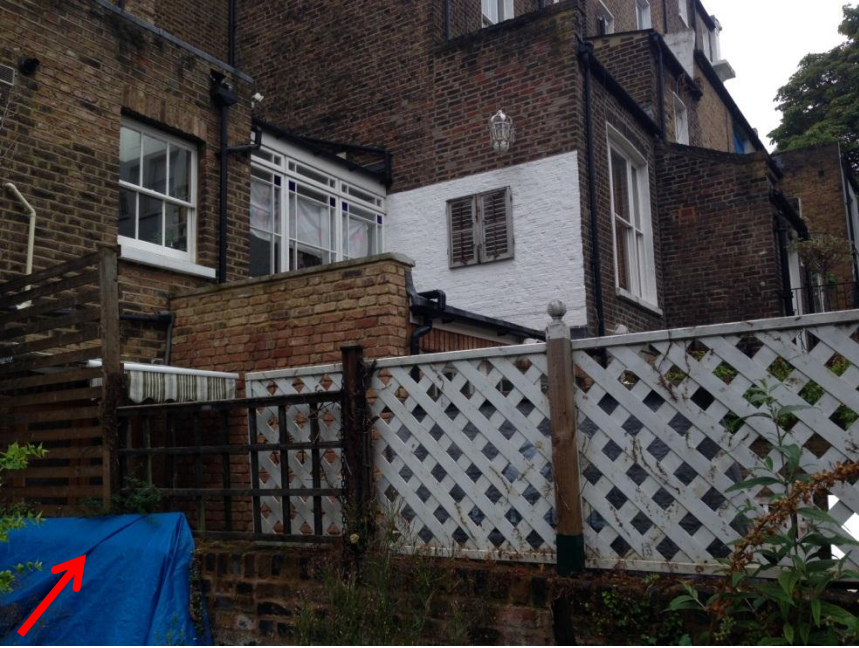
Photo 4: Boundary with 30 Chalcot Road with existing boundary walls.
