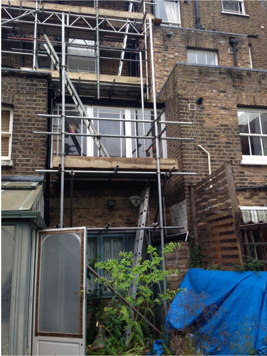
Photo 6: View to rear elevation of host site to upper flats.
