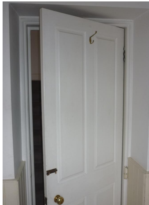
Above left: first floor front room: poor modern door. Lock rail set too high. Original frame.
