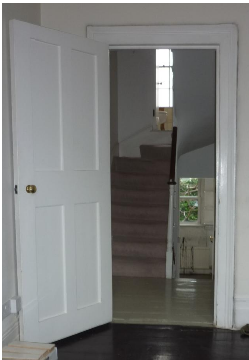
Above left: first floor front room: poor modern door. Lock rail set too high. Original frame.
