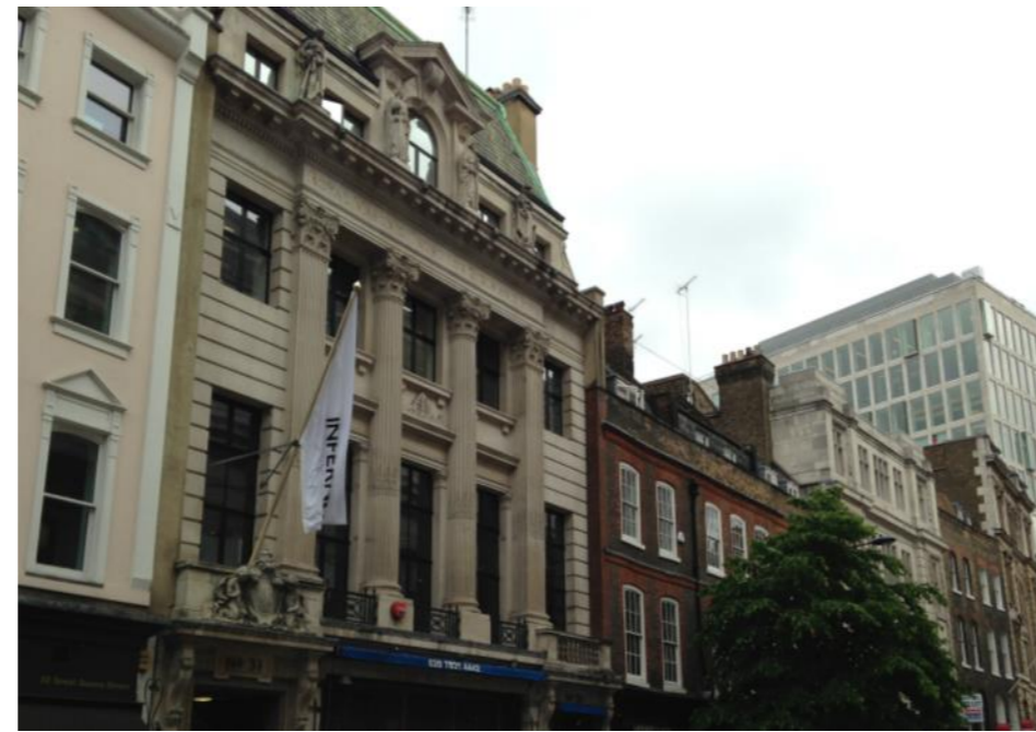
Figure 25: A view of the properties located opposite the property at 34 Great Queen Street. These indicate the nature of the streetscape which is made up of a variety of properties from the eighteenth to the twentieth centuries and which define the character of the Conservation Area in this way.
