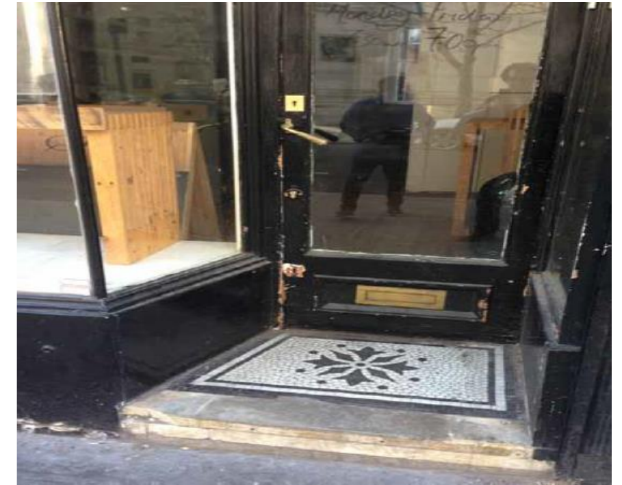
Figure 19: An image of Shopfront entrance double leaf door
