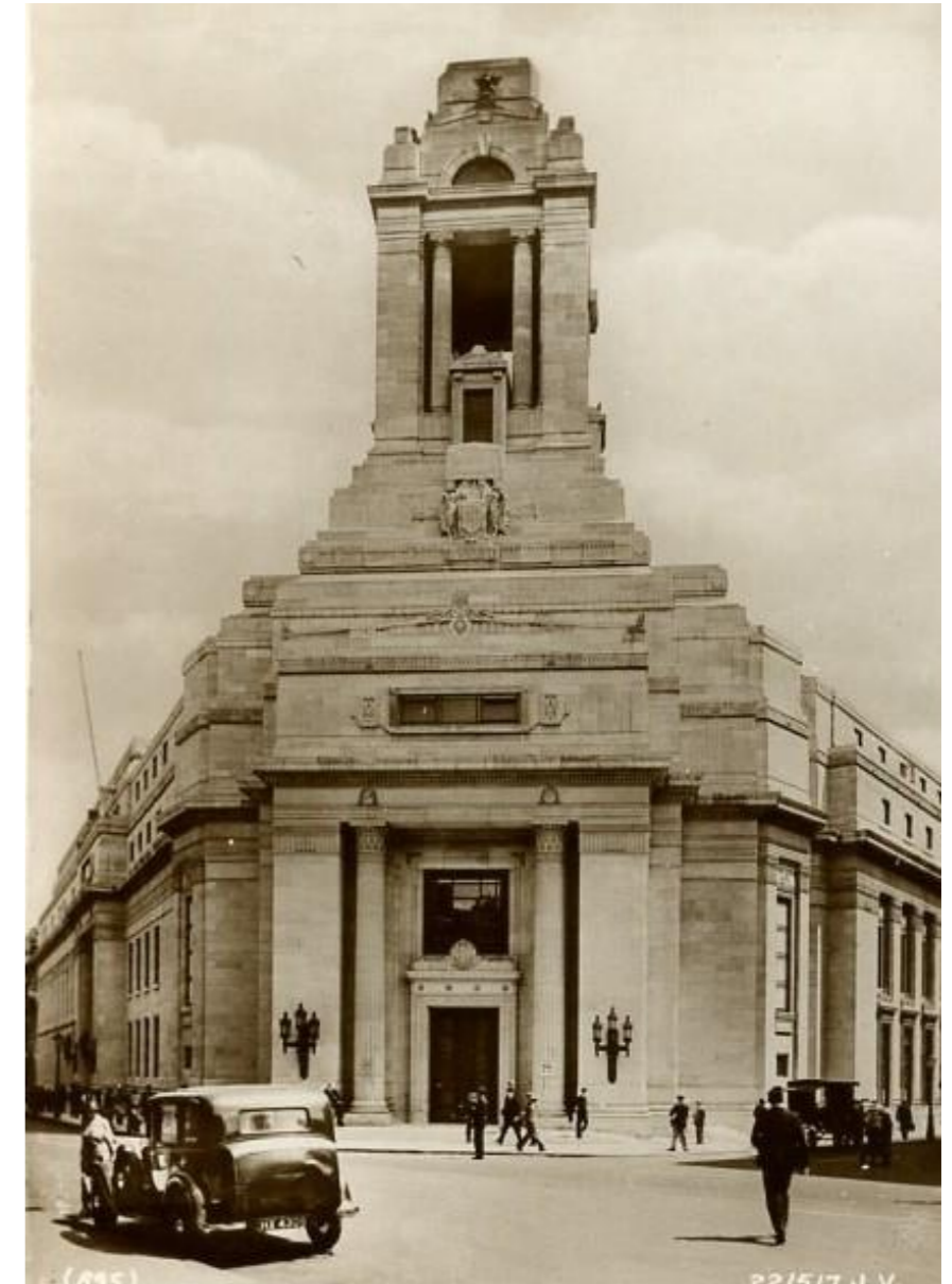
Figure 10: View of the present Freemasons Hall, which dominates the streetscape with its unusual elevations and scale.
