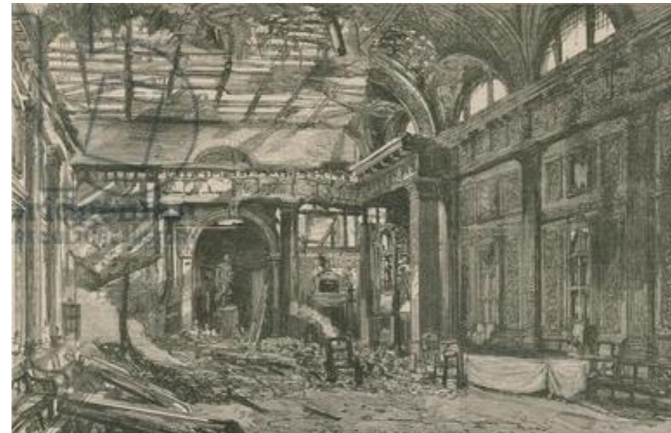
Figure 9: The Grand Hall suffered greatly during a fire in 1883, although it remained in existence until 1932 when it was demolished as a result of structural damage.
