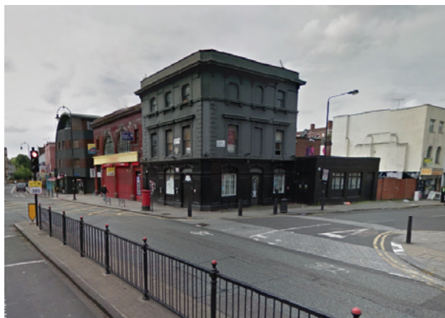
1. VIEW OF SITE FROM KENTISH TOWN ROAD Source: google maps
