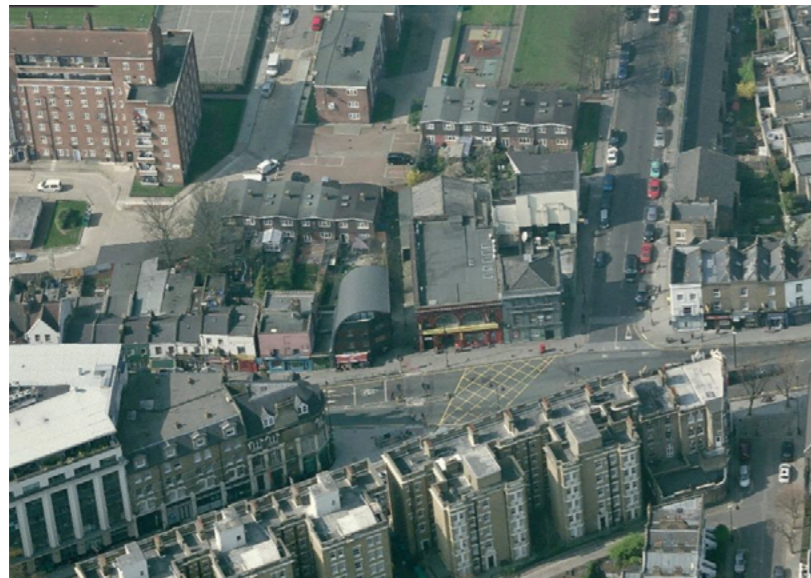
AERIAL VIEW TWO FROM THE EAST- Source Bing Maps
