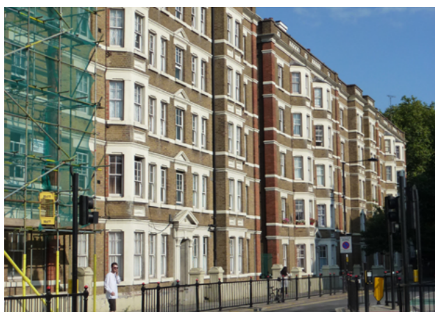
4. VIEW OPPOSITE THE SITE
