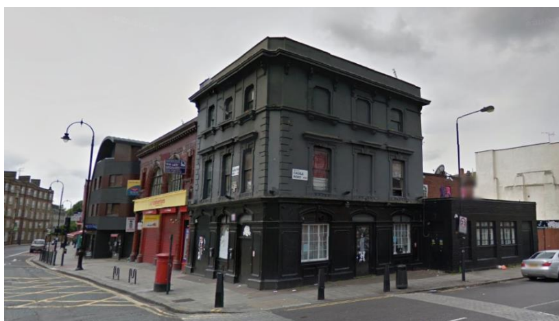
Figure 1: Image of existing building
