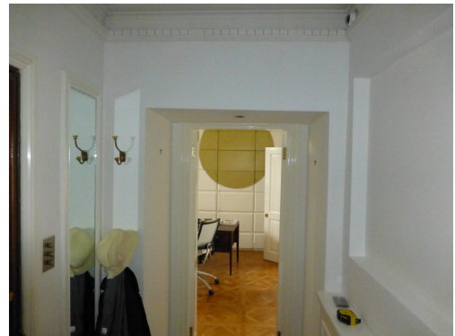
10 Infilled doorway on right of Hallway
