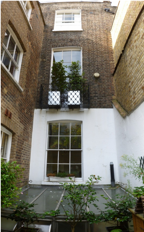
Existing rear elevation of original dwelling.
