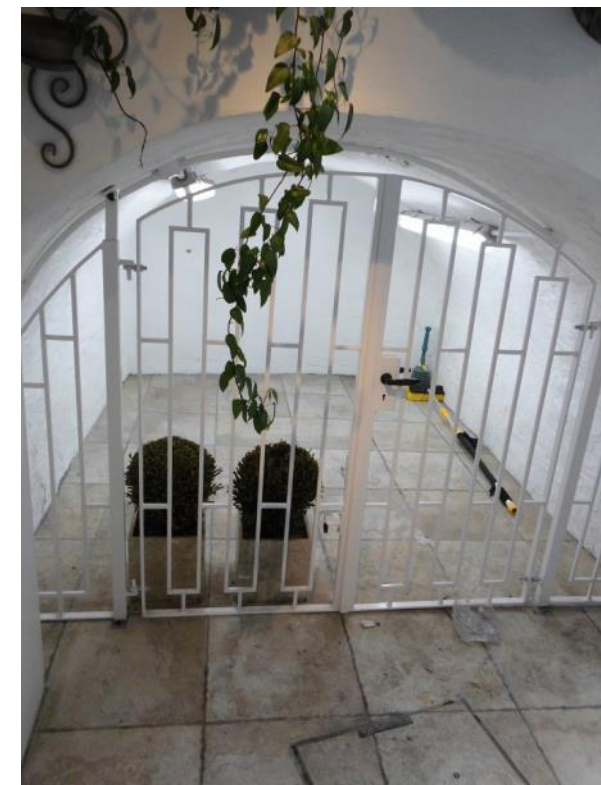
Photograph 8 - View of Existing Vault
