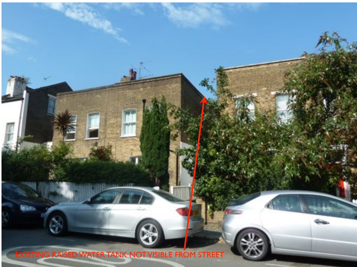
STREET VIEW OF NO 146. FROM NORTH EAST
