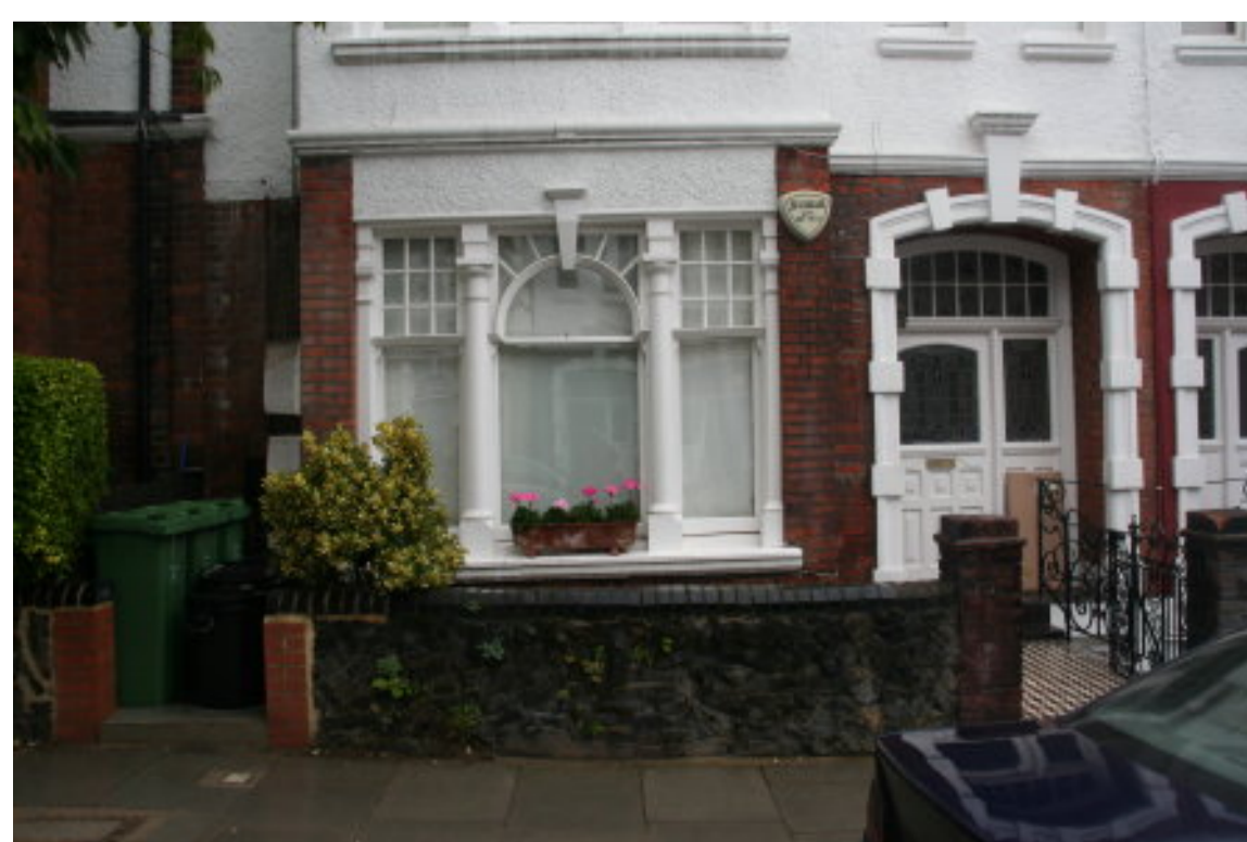
Photo 2: view of the ground floor of 41 Howitt Road. no changes proposed to the boundary wall or to the bin storage area at left.
