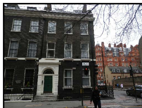
ANTENNA LOCATION VIEW
