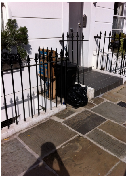
Neighboring Property's platform
