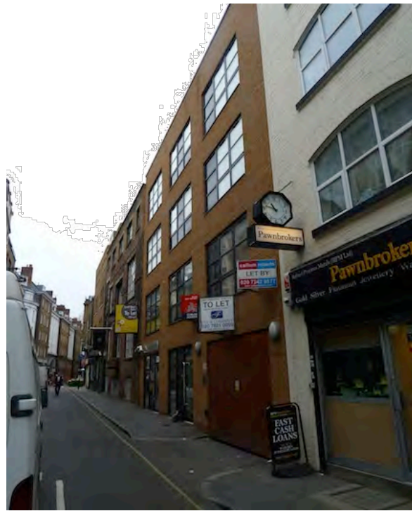
01. Hatton Wall Looking West
