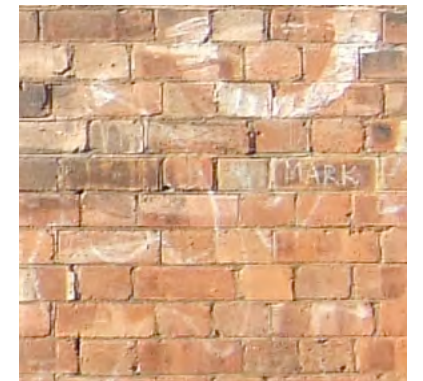
Existing brickwork to Hatton Wall facade
