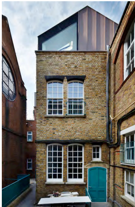
Cladding : Junction of copper and brickwork
