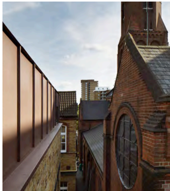
Cladding : Junction of copper and brickwork
