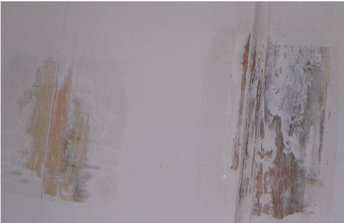
2 No. Paint investigations into original panelling on west wall of ground floor rear room
