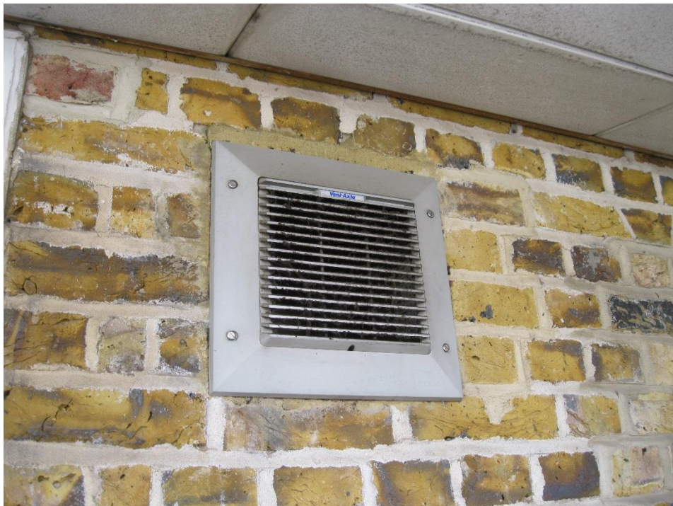
Photograph 4 Larger fan terminal louvre on access balcony, assumed to kitchen, approx. 300mm x 300mm. Some larger examples also present.
