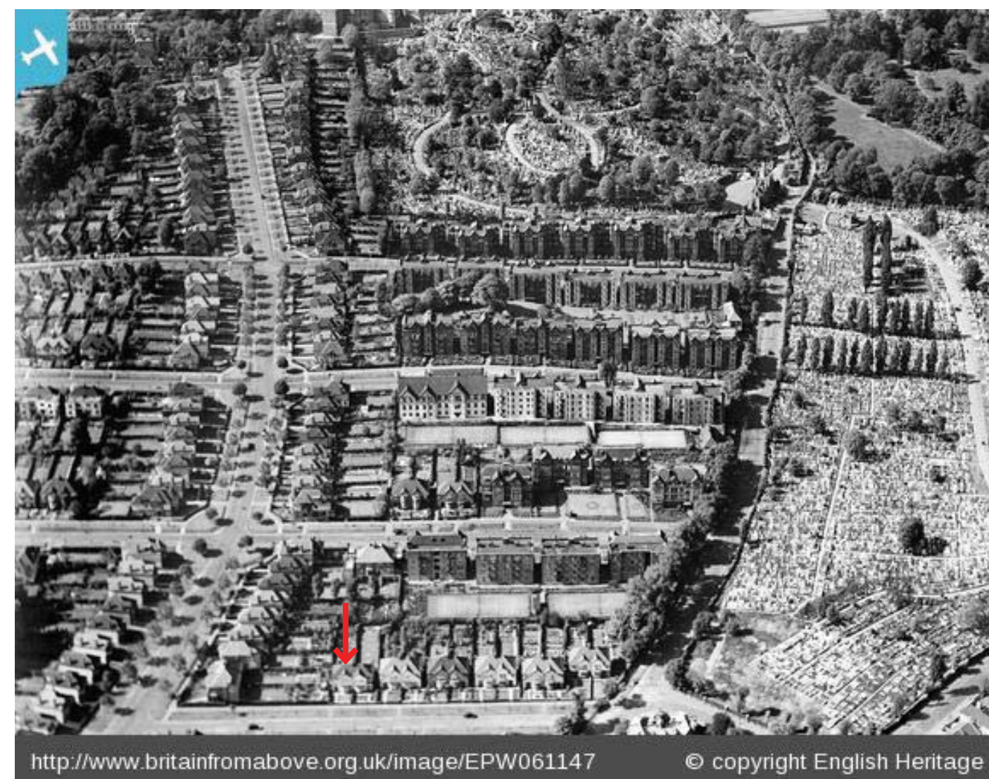
Aerial photograph of Homes Ltd flats at the Holly Lodge Estate and Highgate Cemetery, Highgate, 1939
