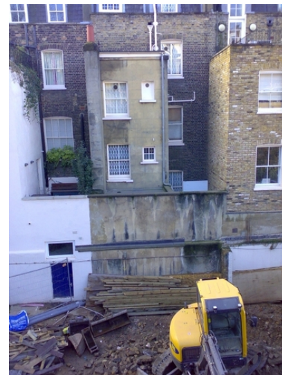
Condition at the rear of the site
