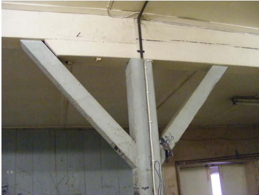
Plate 11: Spine beam, post and braces, ground floor
