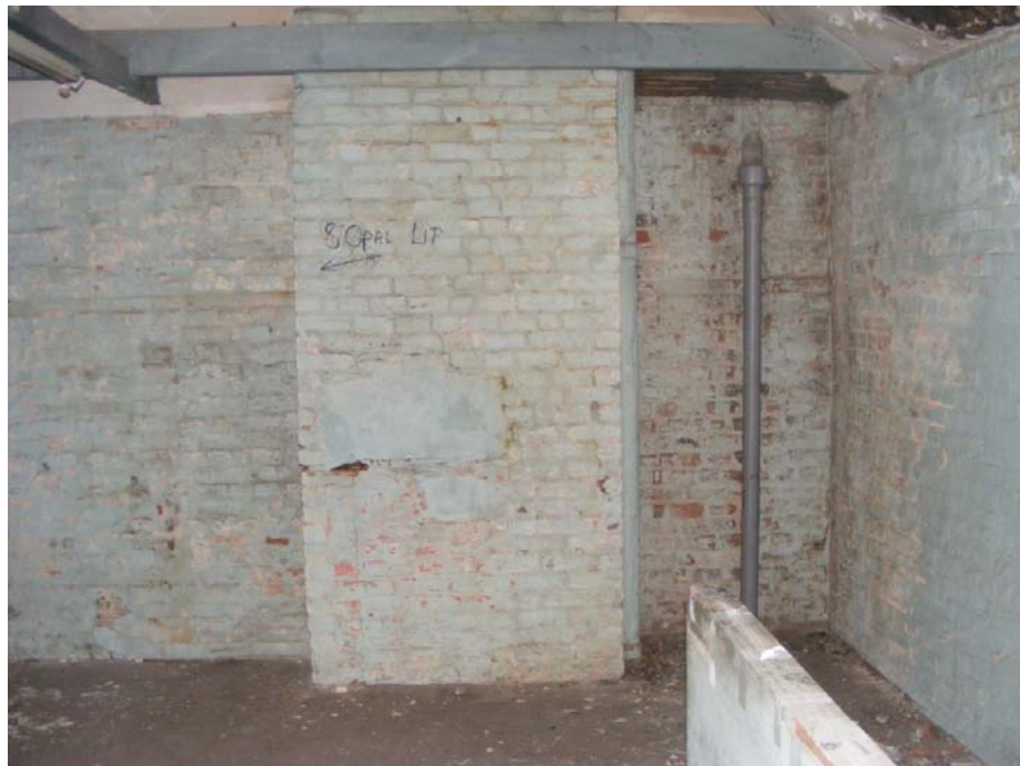
Plate 14: Victorian chimney, blocked, rear wall
