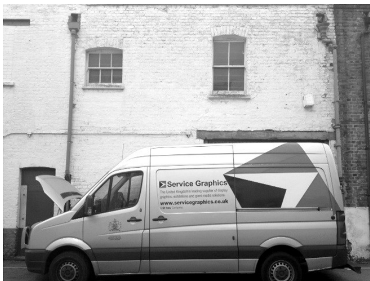
Plate 1 - View of first floor windows at No. 22 Kings Mews
