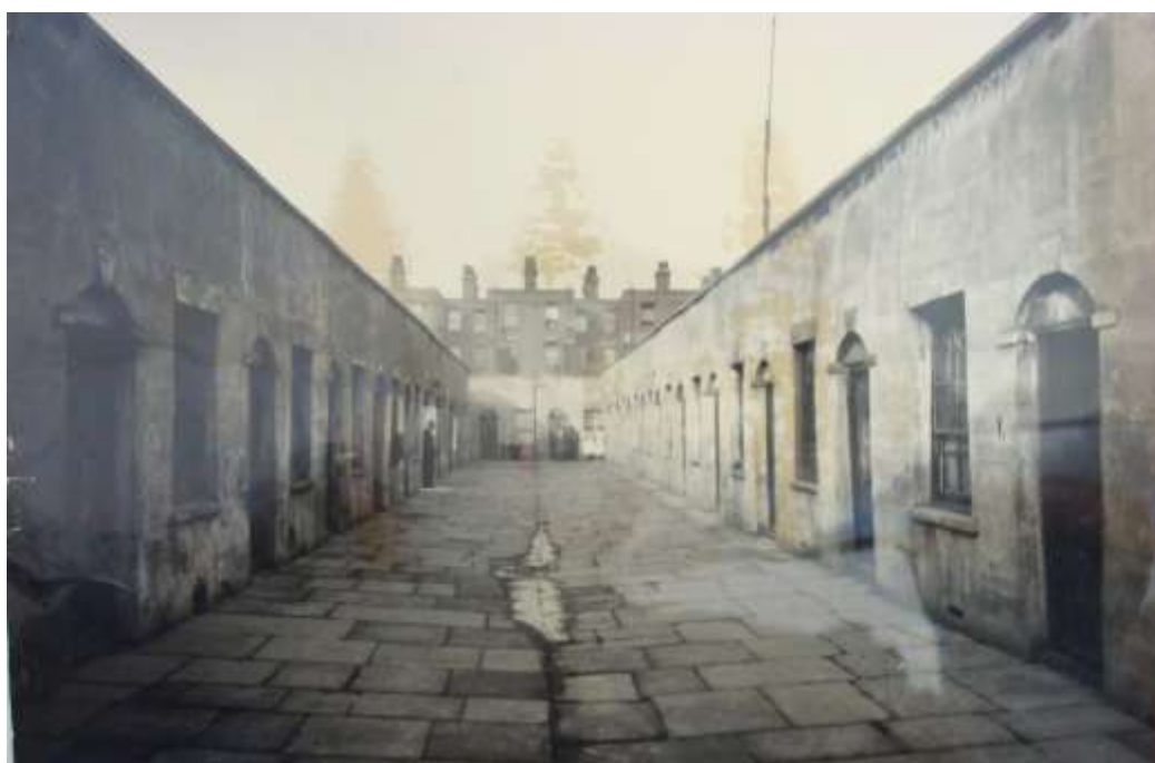
Figure 7: Equity Buildings, Looking North, 1928
