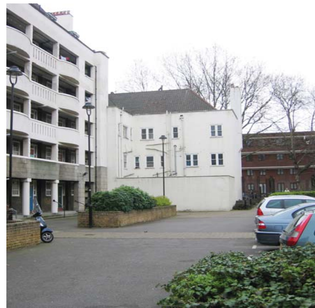
2. View from courtyard looking West
