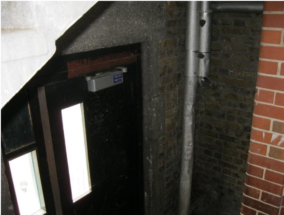
Photograph 20 Communal entrance – ground floor south west
