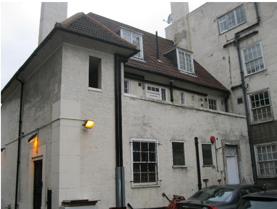
Photograph 4 Rear elevation retail unit 16/18 Weirs Passage
