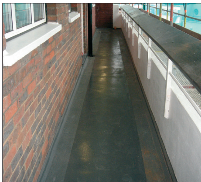
Tordeck™ on-site in London, UK.
