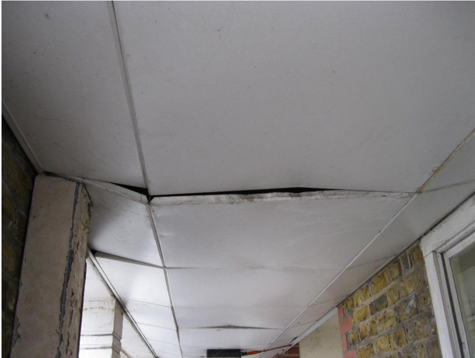
Photograph 22 Access balcony suspended ceiling
