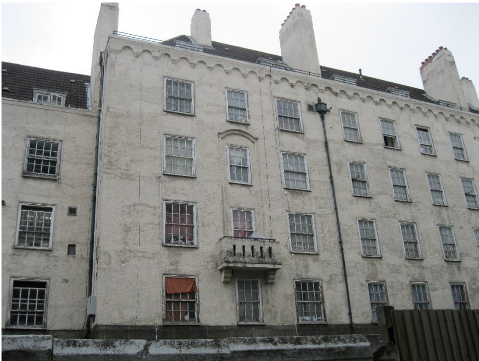
Photograph 2 South East/Rear elevation – part Weirs Passage
