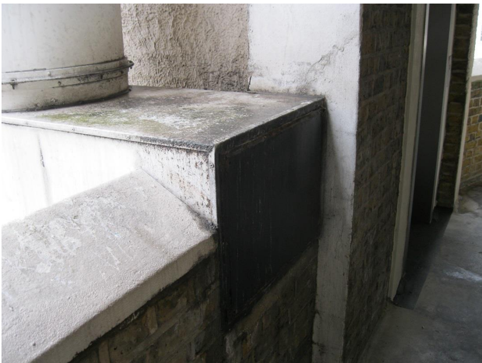
Photograph 23 Access balcony refuse chute
