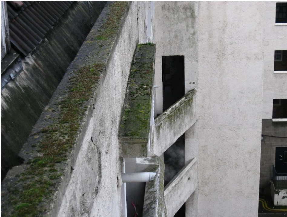
Photograph 14 Render North west side, blown
