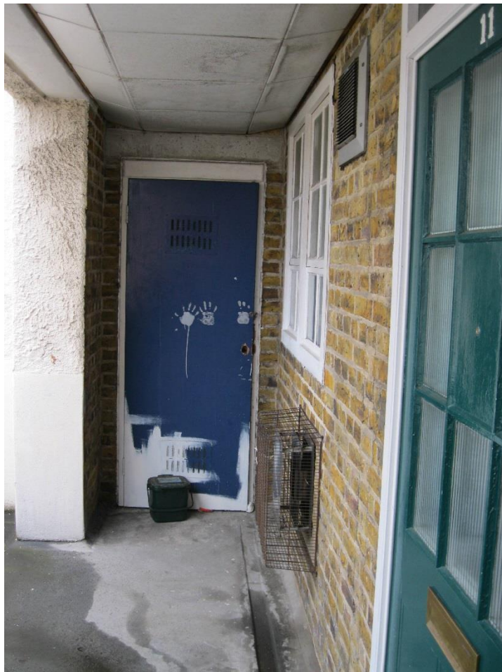
Photograph 17 Access balcony flat entrance door No 11 and store door
