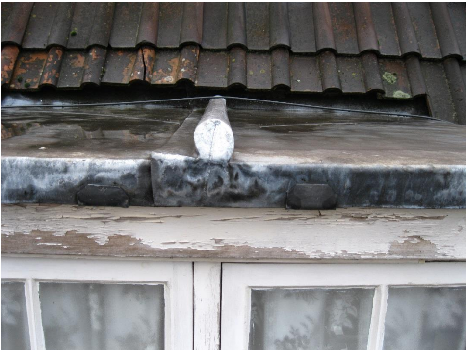
Photograph 12 Dormer roof and window
