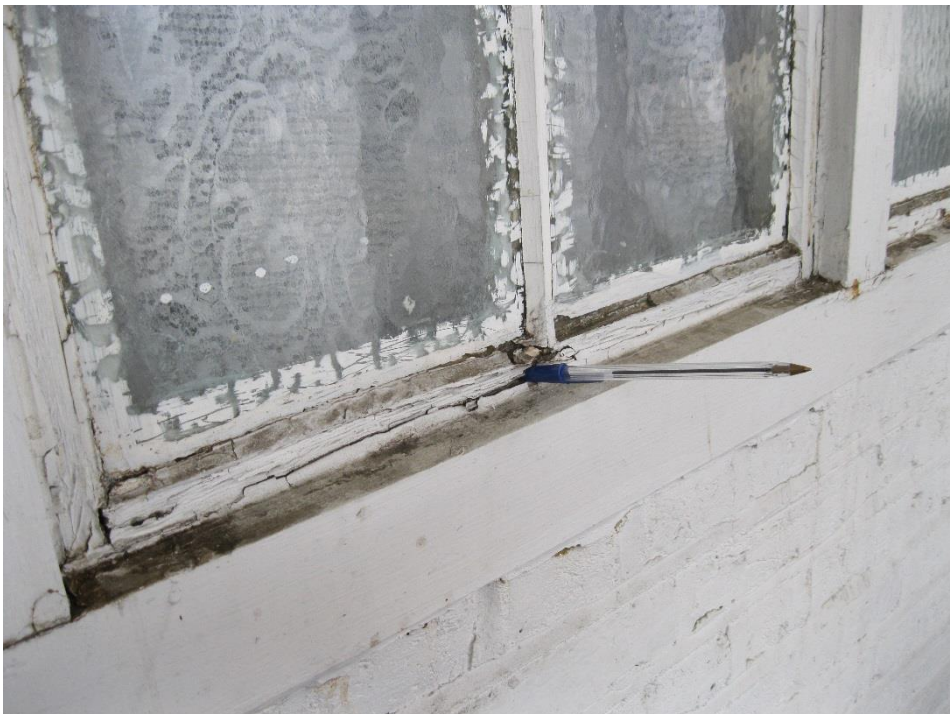
Photograph 16 Access balcony window – flat 21
