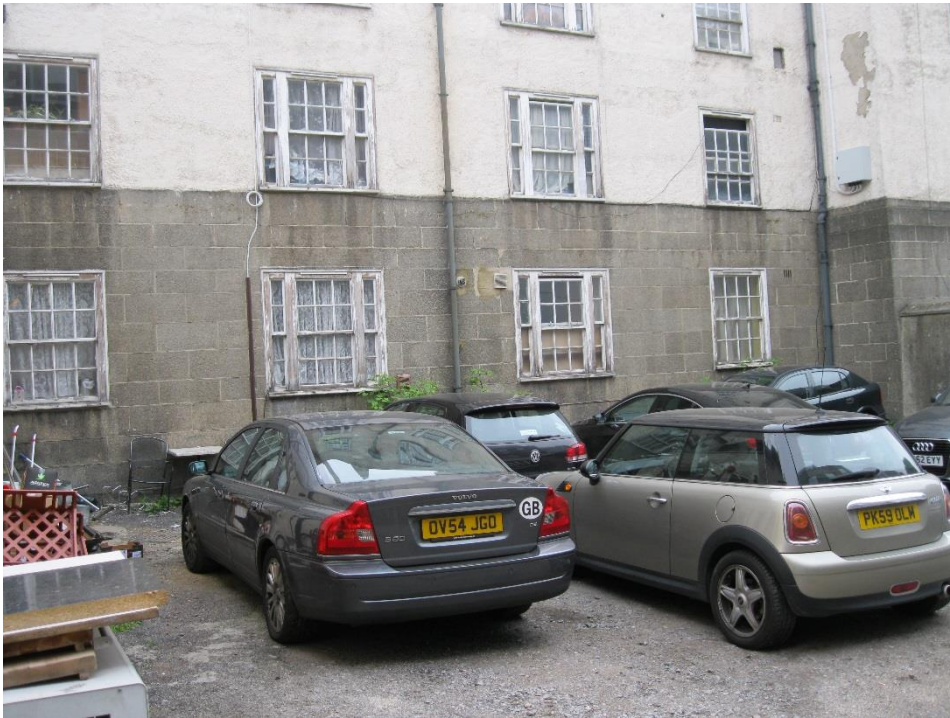
Photograph 3 South East/Rear elevation behind retail unit 16 – part facing Weirs Passage
