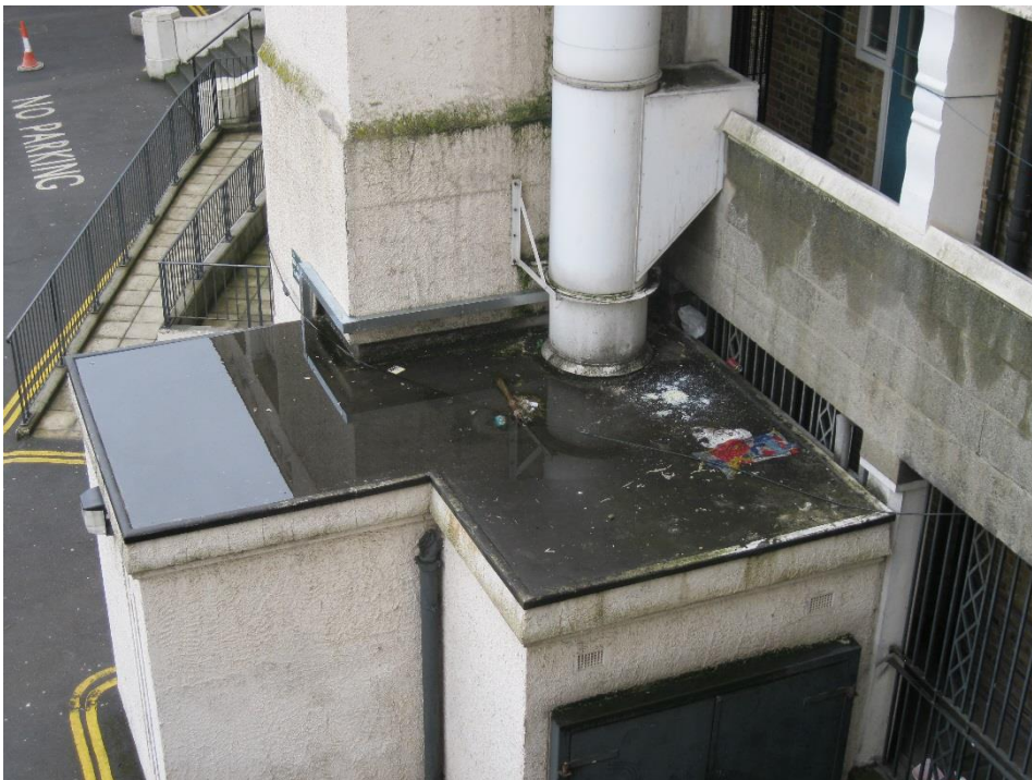
Photograph 19 Low level flat roof
