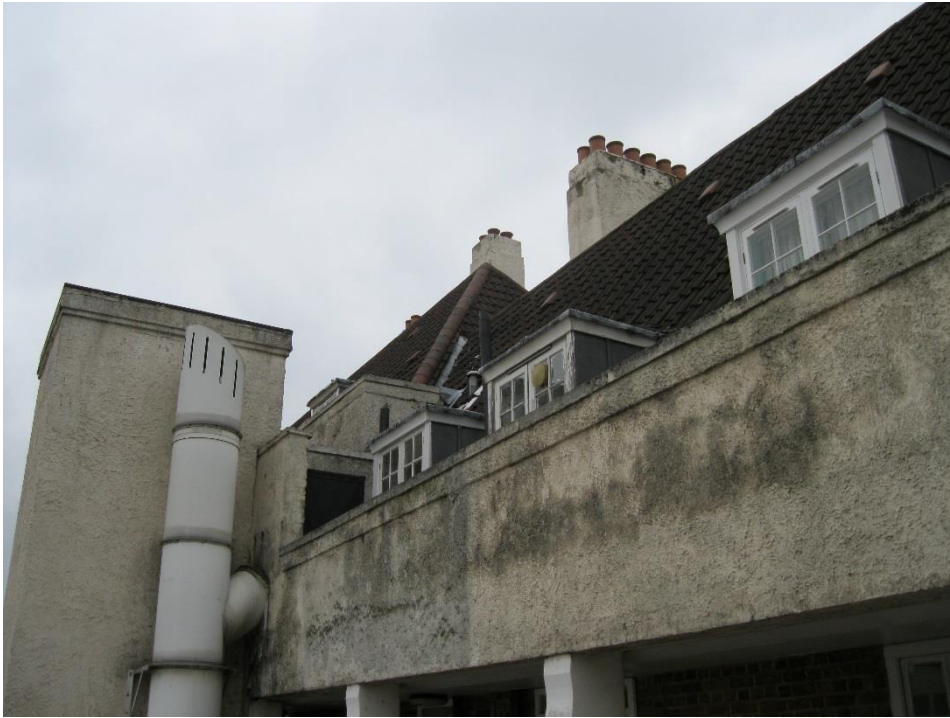
Photograph 1 Front Elevation (Part) Courtyard
