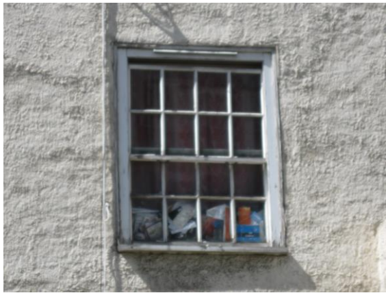
Existing sash window in 1 -21 Levita House
