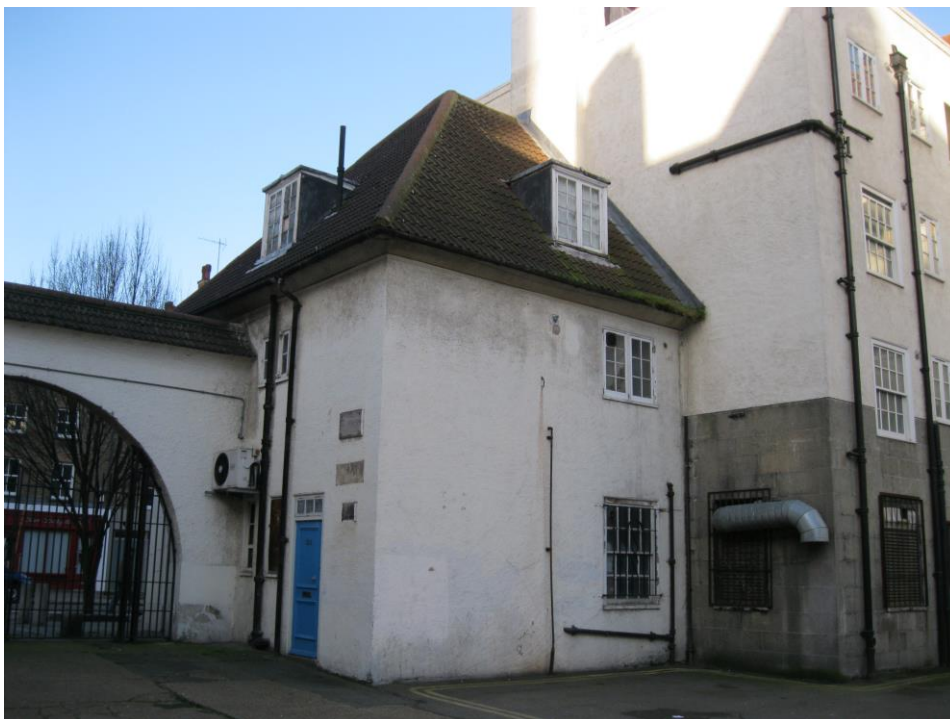
Photograph 25 No 28 wing and arched entrance to courtyard adjoining part Levita House already refurbished
