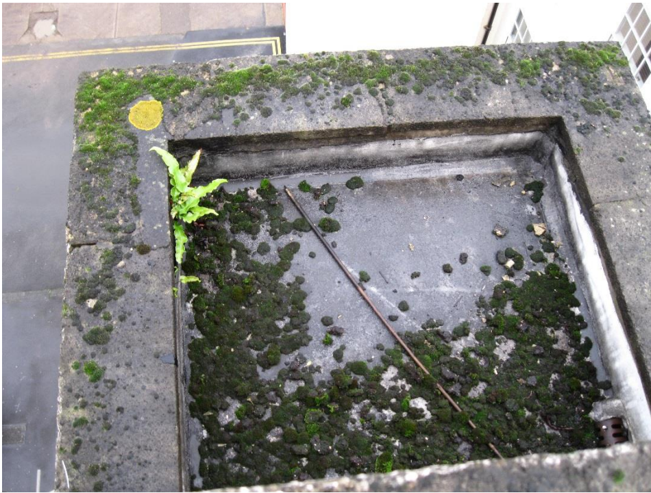
Photograph 15 Flat roof, north end
