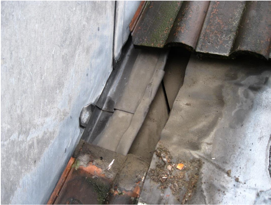
Photograph 11 Secret gutter and dormer detail
