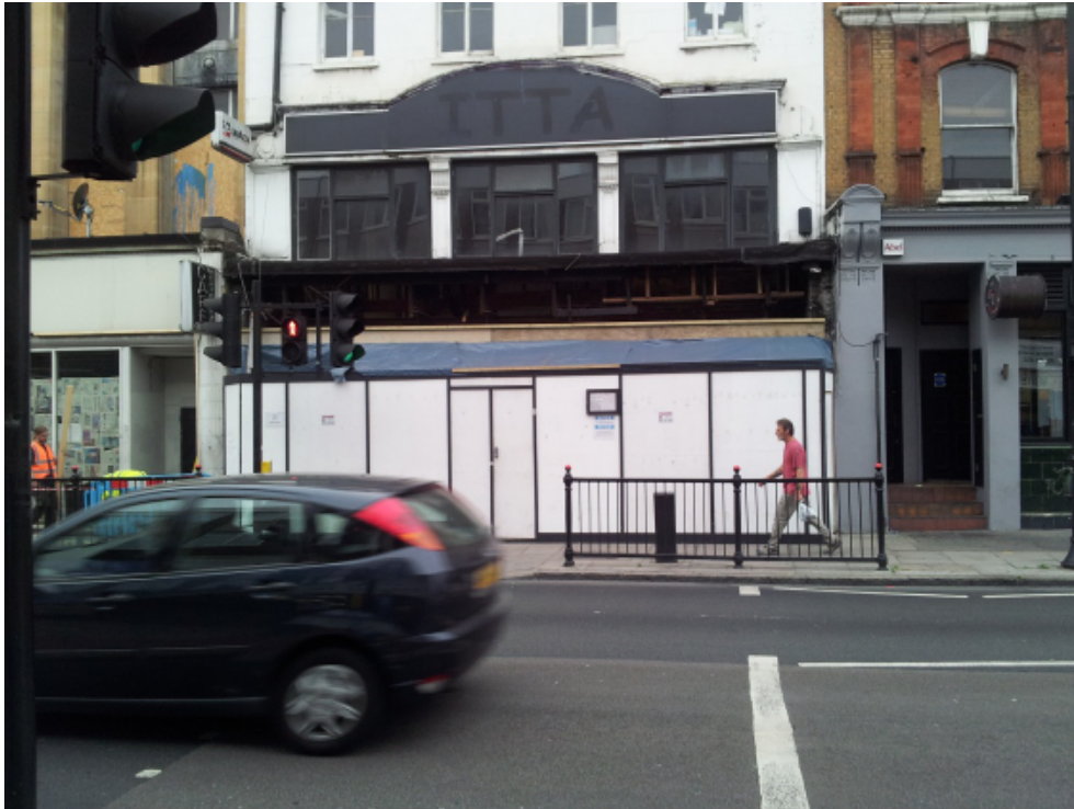
Above: Front elevation of the application site at 225 Kentish Town Road
