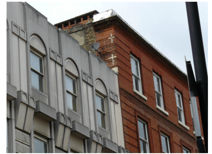
existing junction between the buildings
