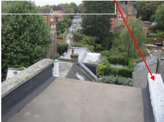
Photo 1 View facing to rear of No 29
