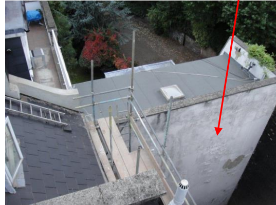
Photo 6 View facing No 27 and Air Duct
