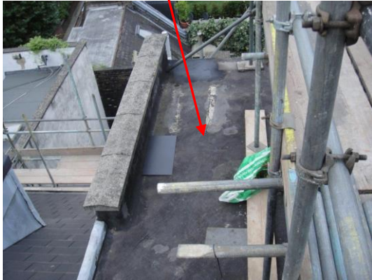
Photo 5 View facing Daleham Mews
