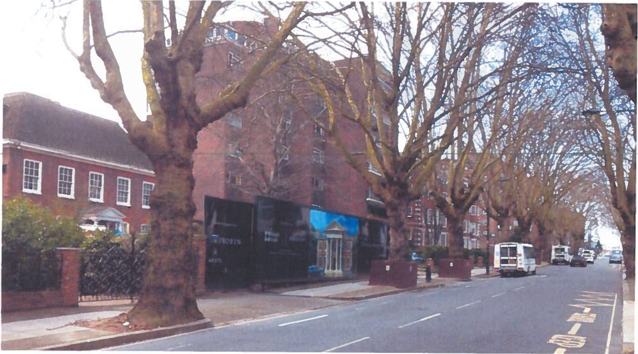
Photograph 1: Box hoarding around plane trees along Avenue Road
