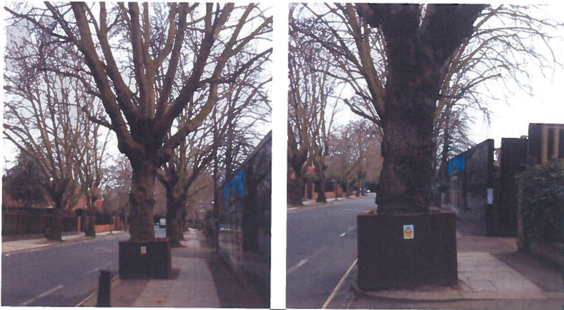
Photographs 4 & 5: Box hoarding around plane trees T2 and T3
