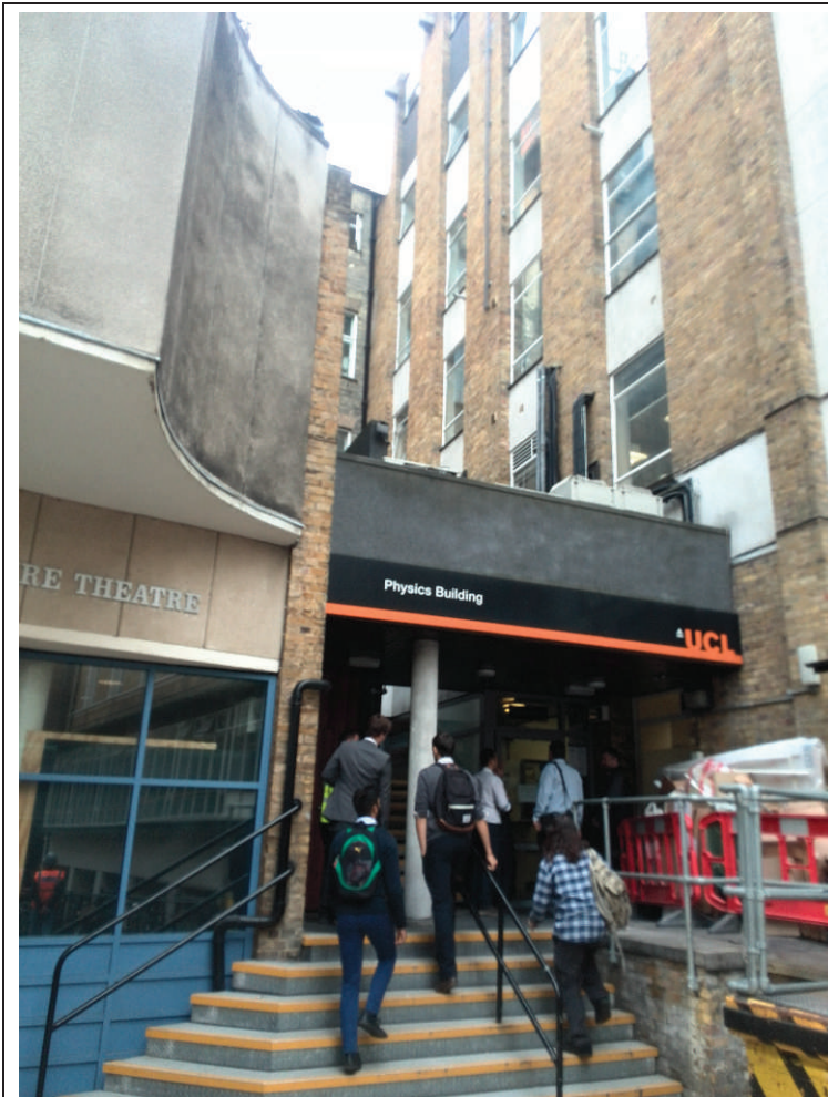
View facing east towards the Physics Building entrance showing the roof plant area above the entrance doors. Photograph taken on the 26.09.2014.
