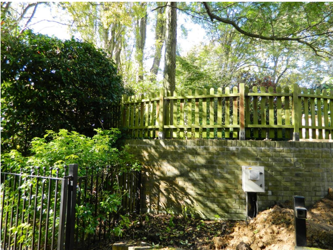
Figure 3. Retaining wall 1.3 m high and 1.7 m away from the trunk of T5 restricting root growth
