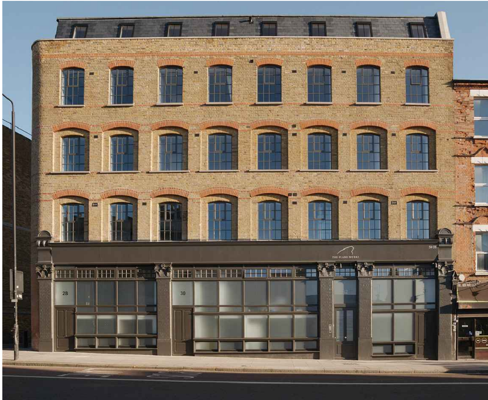
Precedent Image - Refurbishment of Piano Works on opposite side of Fortress Road
