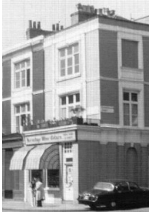
1972 Hermitage Wine cellars
