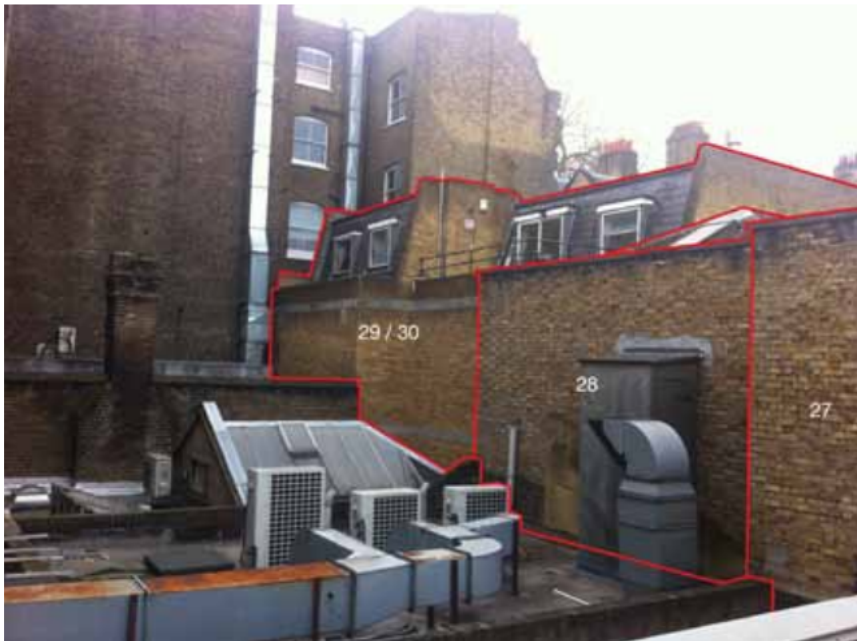
Properties to rear at Kings Mews (viewed from 41 Gray's Inn Road)
