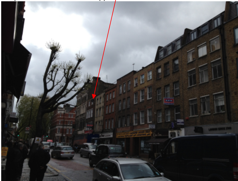
Gray's Inn Road elevation – prior to work starting on adjacent sites
