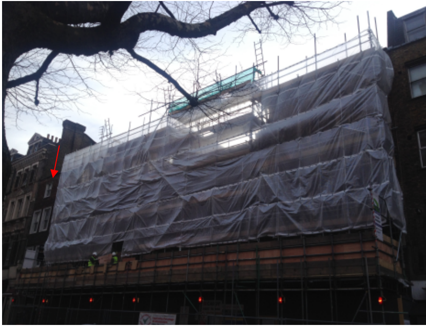
Gray's Inn Road elevation – works underway on adjacent site
