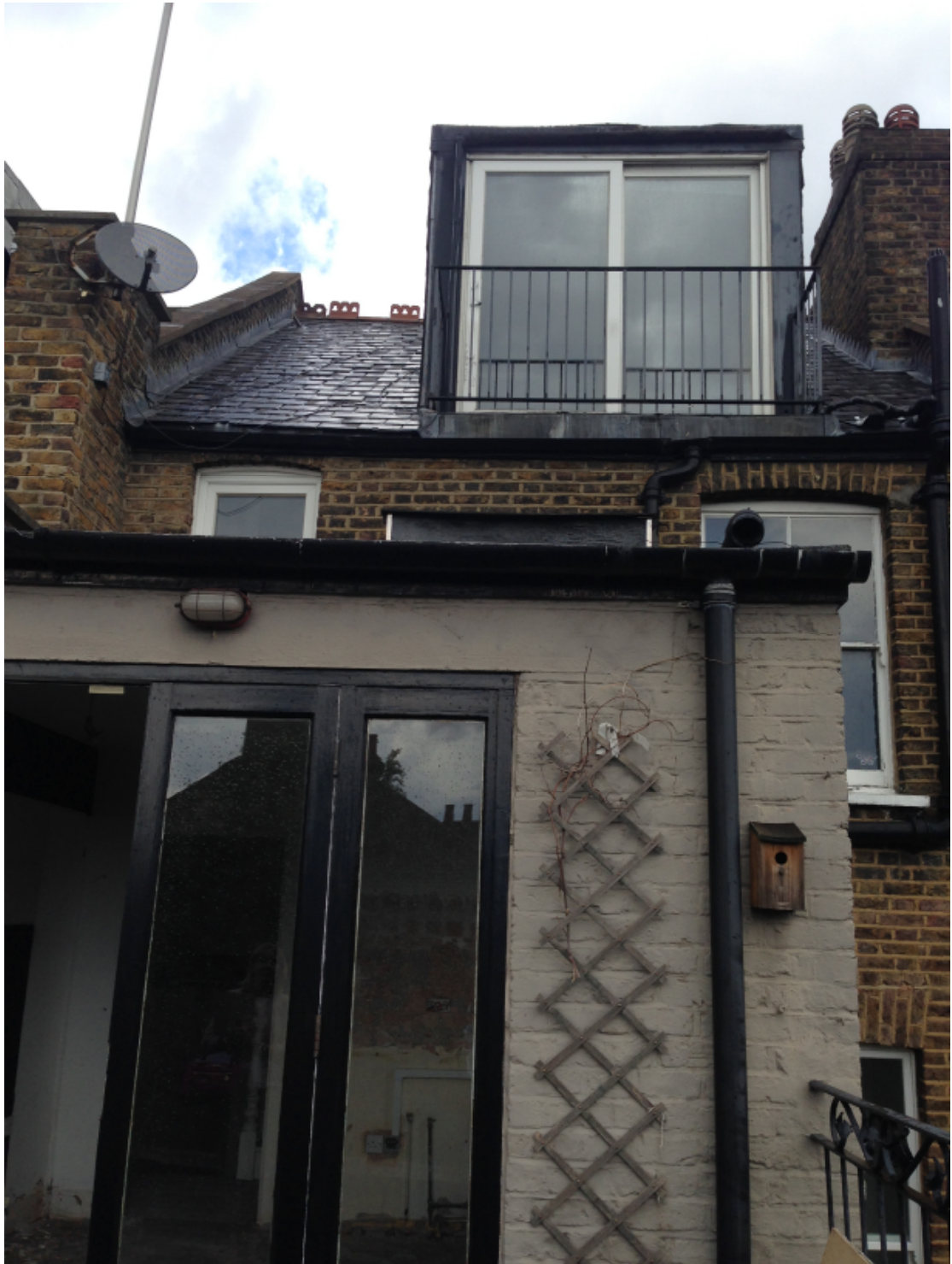
Rear elevation at 2 nd floor level
