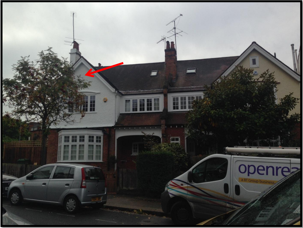
Photo 2: Showing existing front rooslope and arrow showing location of proposed 'bullseye' window.
