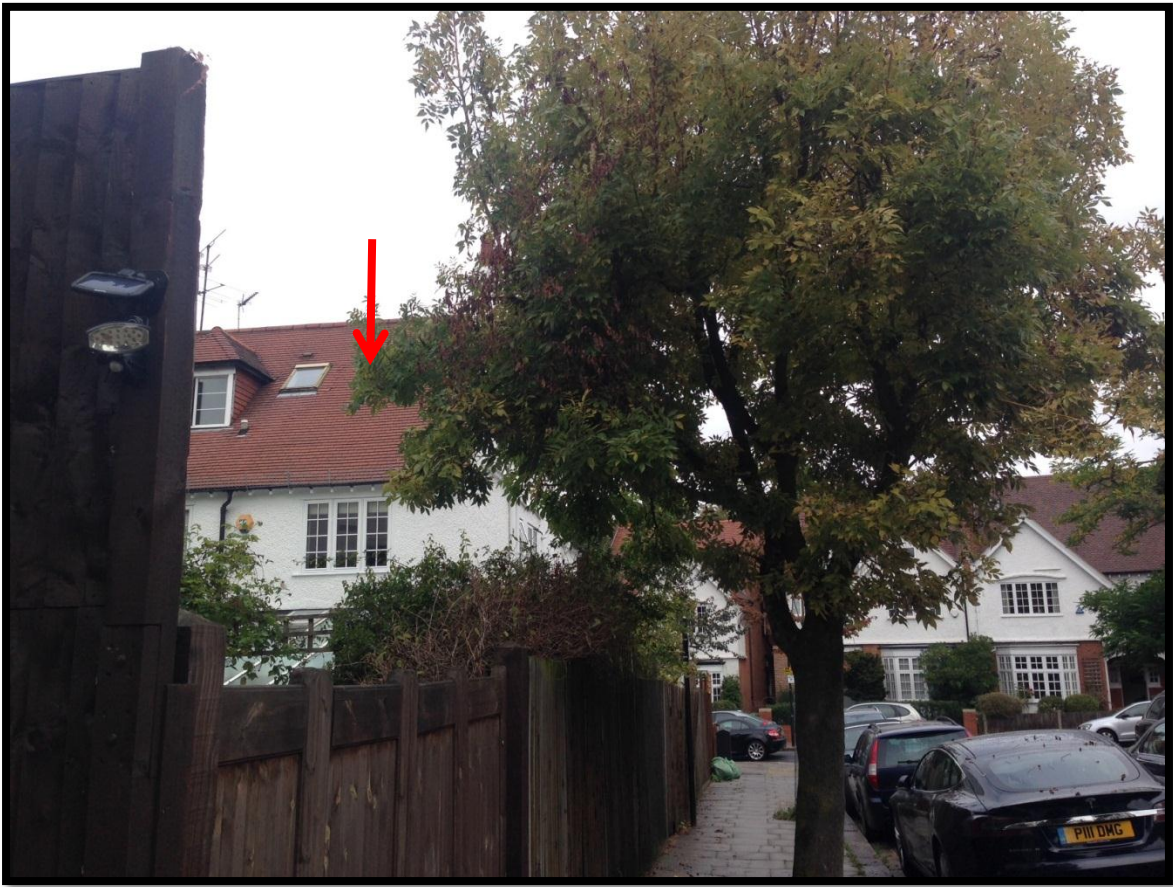
Photo 4: View to rear elevations of host site from Clorane Gardens with arrow showing location of proposed rear dormer
