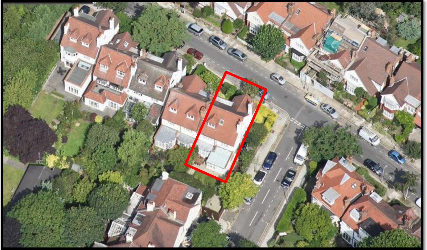
Photo 1: 6 Briardale Gardens – shows existing rear dormer.
