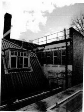
First floor (W); close window (5M); sky to be lost
