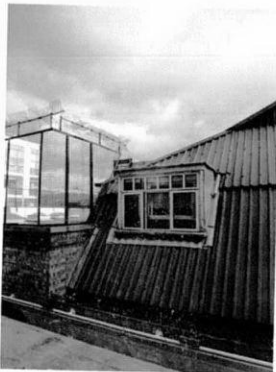
First floor (E); close window (5M); sky to be lost
