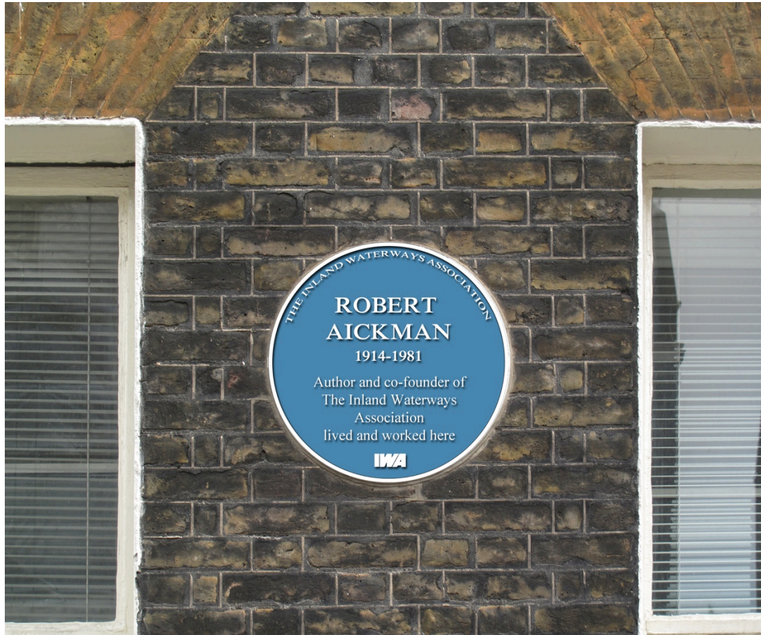
Proposed location of the plaque between the ground floor windows
