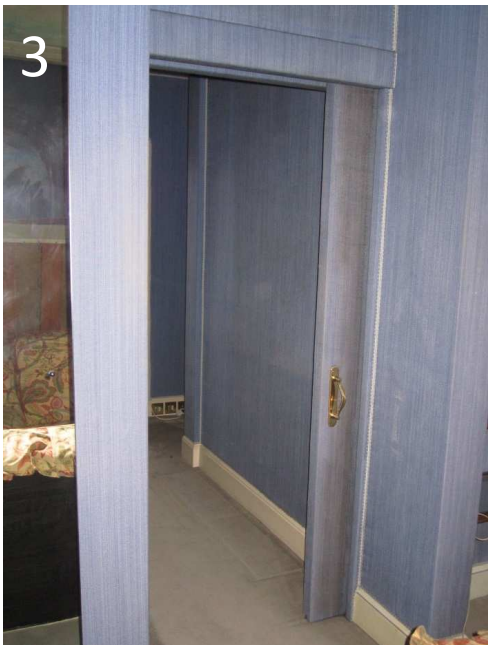
3 View looking at the entrance door leading to the dressing room and master bathroom
