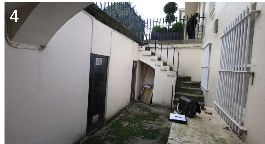
4 Lower Level Courtyard, Giving access to underground vaults.
