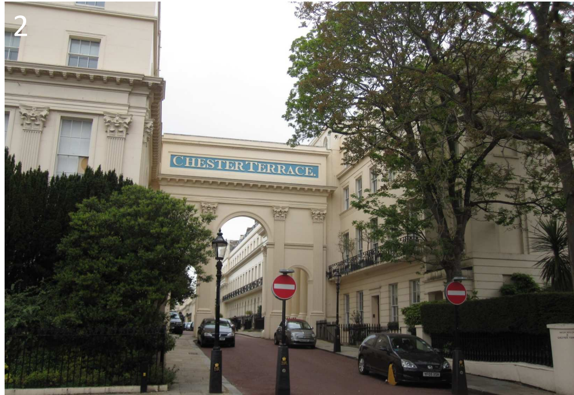
2 Looking at one of the 2 Corinthian arched entrances to Chester Terrace.
