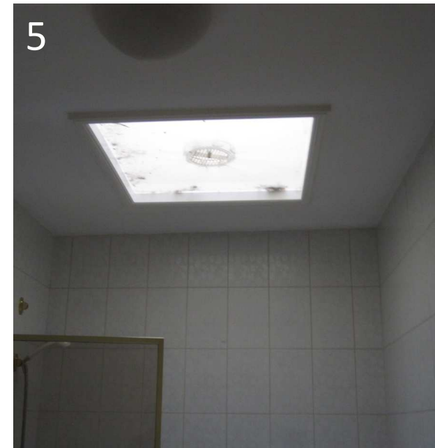
5 View from the bathroom looking at the roof light.
