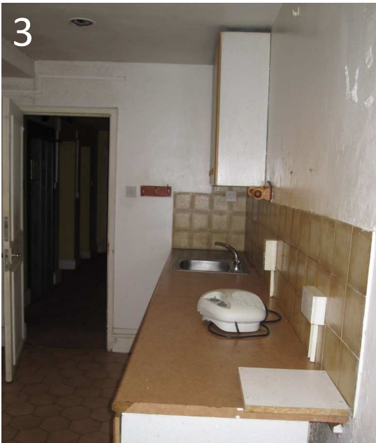
3 Staff kitchen, looking through into the hallway.
