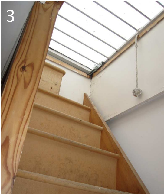
3 View looking up towards the roof access hatch
