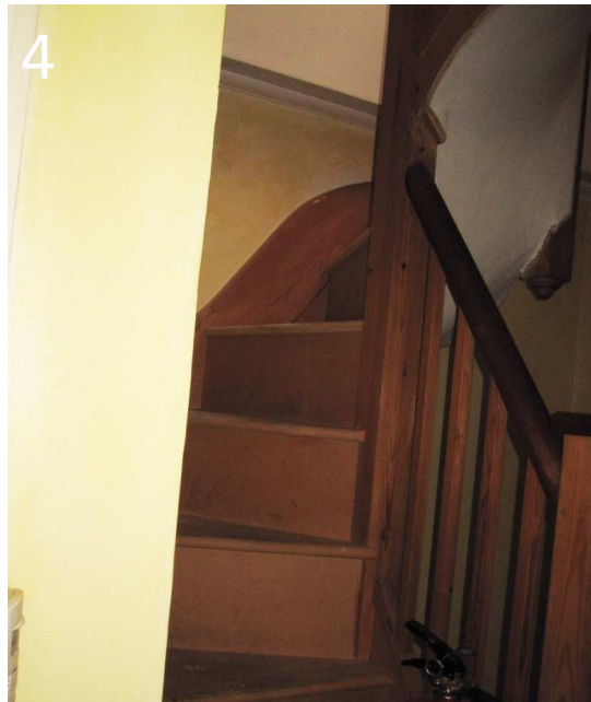
4 View from the third floor looking up the roof access stair.
