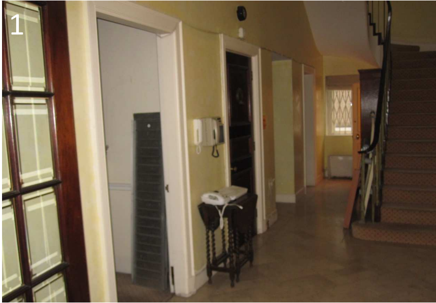
1 View from the ground floor entrance lobby towards the lift and main staircase.
