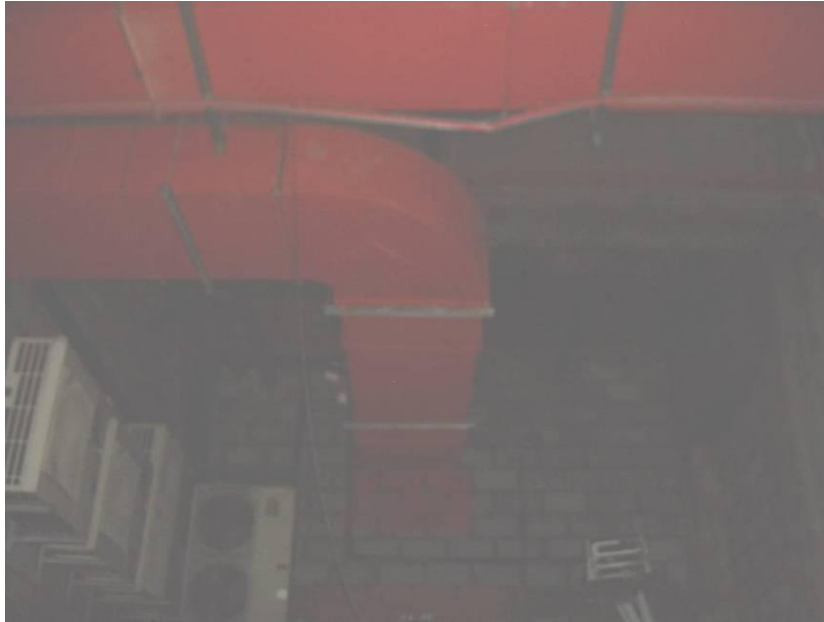
P11 – Service Road Existing LEV Ducting
