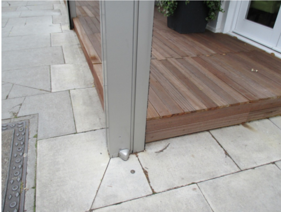
Photograph 2: The deck is 150mm high and is fixed to the frame which in turn is fixed to the floor.
