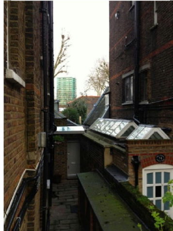
VIEW OF GAP BETWEEN NOS. 76 & 74
