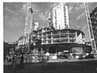
Westminster Park Plaza, London Construction of new luxury hotel by top-down method incorporating 4 basement levels
