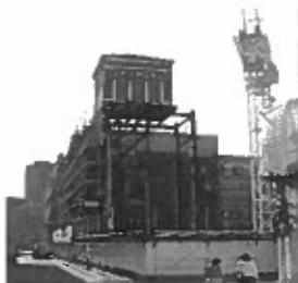
Whitefriars, London Façade and water tower retention prior to basement construction
