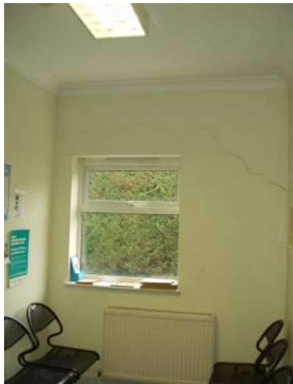
PHOTO 4 : Typical Internal Fracture Damages
