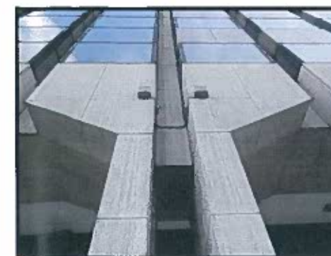
ANTENNA LOCATION VIEW
