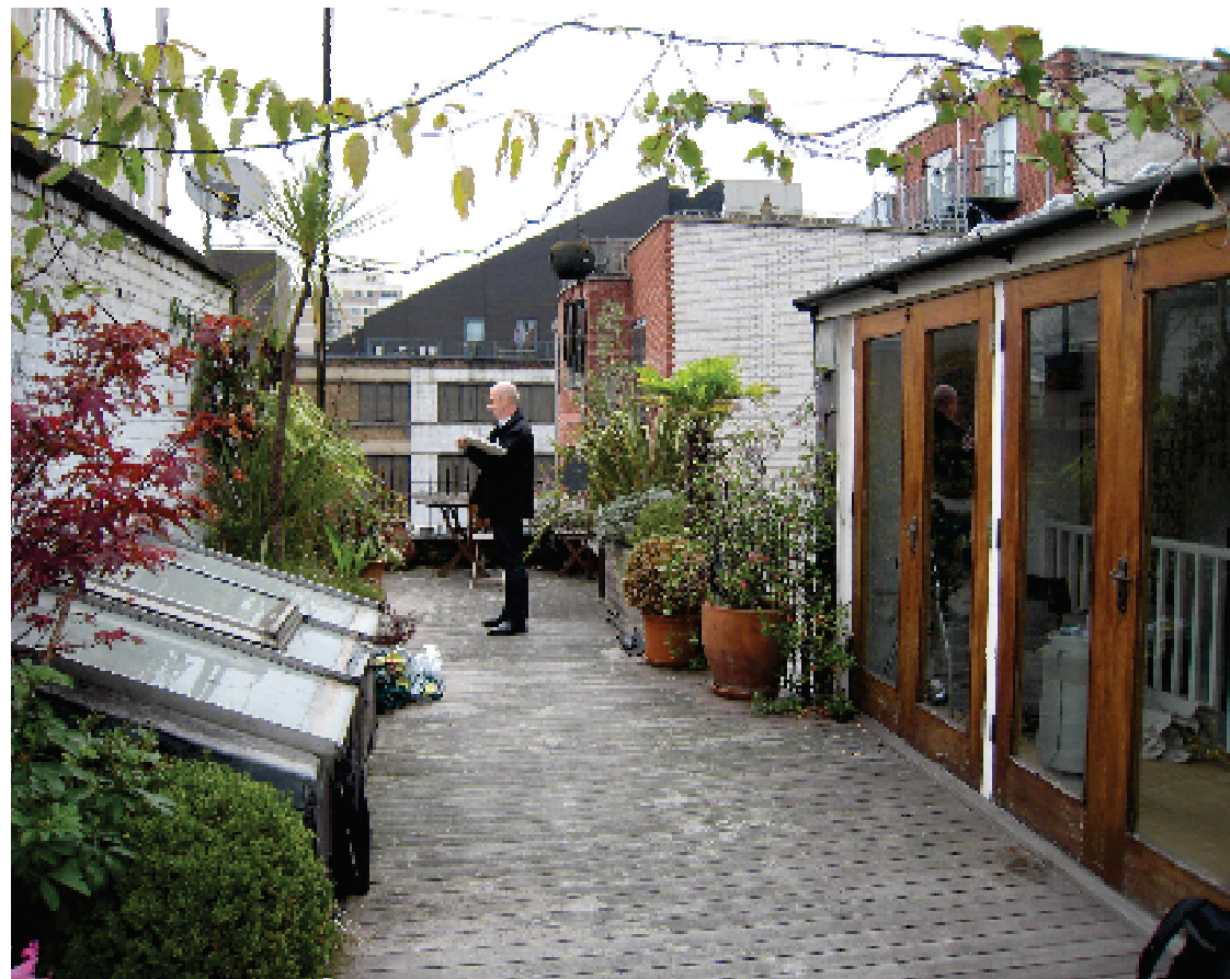
View looking rearwards across space where proposed extension will infill with glass.
